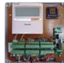
PCB, Power trans, Terminal block
