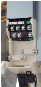
Bigger working space for wiring connection.
