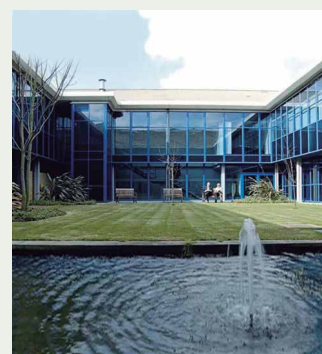
NHS Canford house clinic, Bournemouth, UK. VRF
